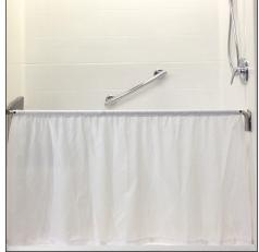
**Step 9: Install curtain.** Thread top of curtain through telescoping rod to complete the installation.
