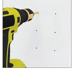
**Step 3: Drill holes.** Determine correct size drill bit for the fastener to be used. Always use a drill bit with countersink head to avoid risk of screw cracking or chipping finish (Tile, marble, granite, acrylic or Fiberglass, other).
