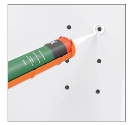
**Step 4: Apply Caulk.** Always apply caulk in a circular pattern around each hole drilled to prevent water migration into the wall cavity. Use a premium clear silicone adhesive caulk.
